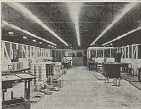
Above: Multi rows of 500 W. Cosmos tungsten lamps in dispersive fittings in an engineering shop.
