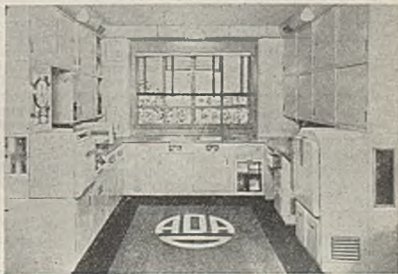
General view of the aluminium kitchen
