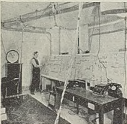
Temporary control for S.E.E. and E.E. areas during construction
