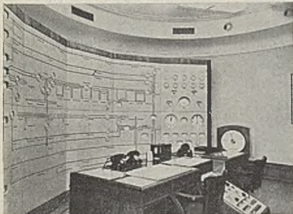
Area loading control room
