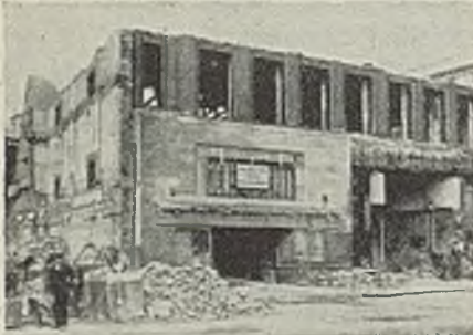
Exterior view of the national and area control centre during construction
