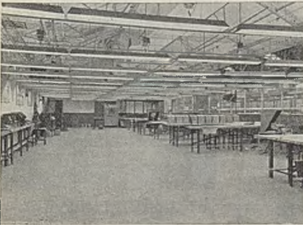
B.T.H. fluorescent lighting in an assembly department
