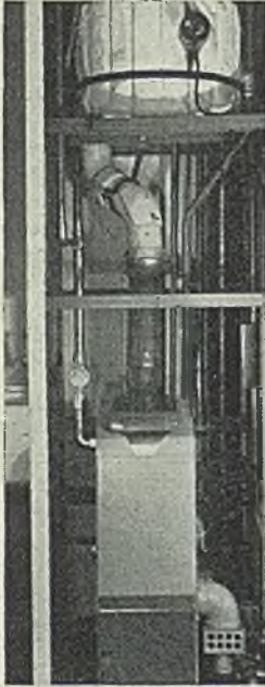
The hopper boiler, showing on the right the automatic damper. The thermostat is just behind this. The valve controlling the flow of water is on the pipe at the side
