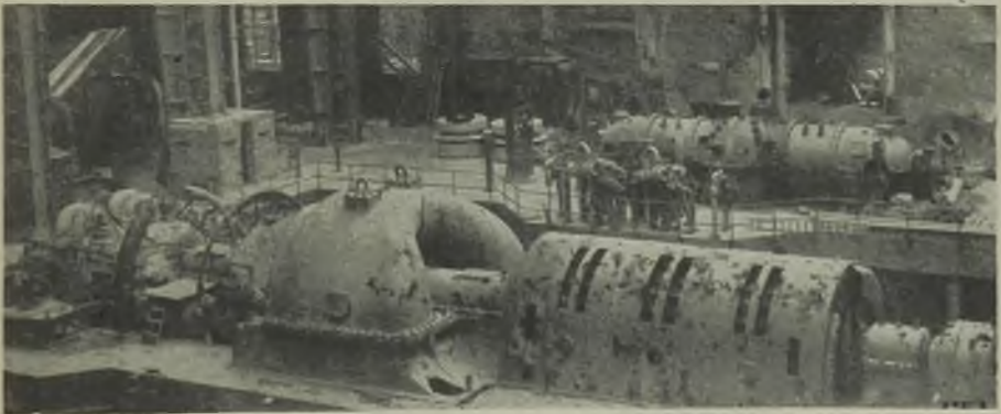
How two of the turbines at Fulham looked when the debris had been cleared away after a bomb had exploded between them
