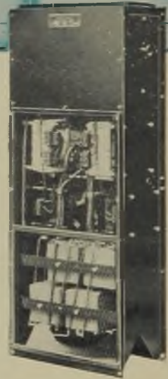
Typical 1,200 watt "Westat" supplied to the Southern Railway for floating batteries
