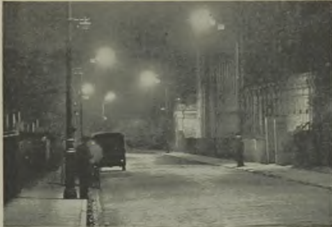
Demonstration street lighting at St. Albans employing 140-W sodium discharge lamps
