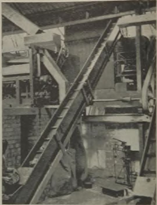
Feeding the sunflower heads into the conveyors leading to the de-seeders
