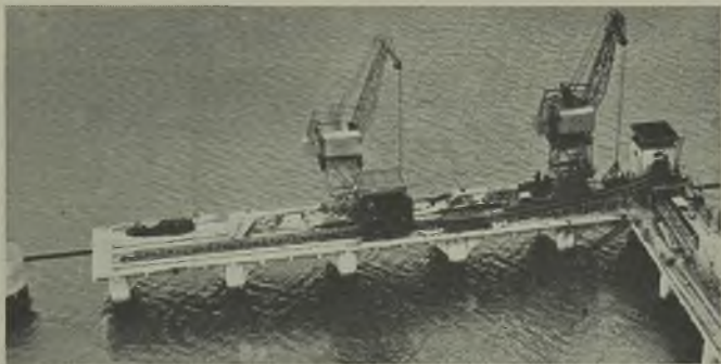
Reinforced concrete jetty showing two coal-handling cranes and conveyor system
