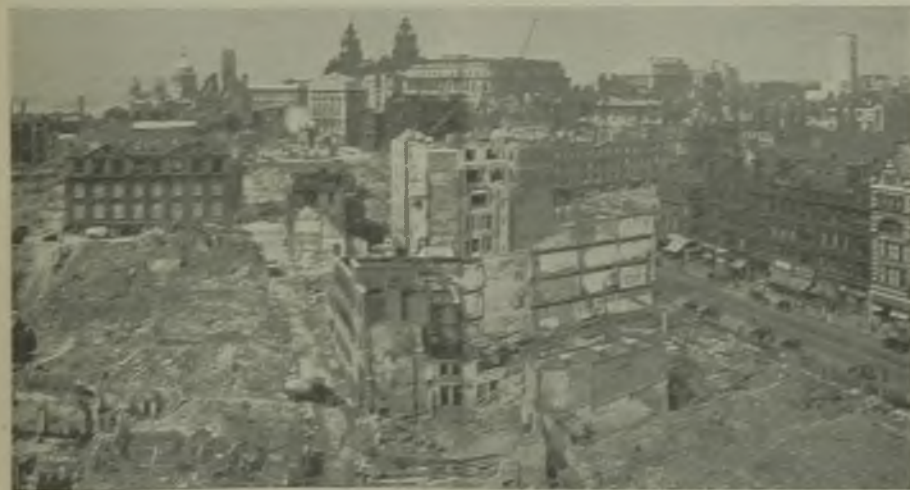
One of the most devastated areas. Note the undamaged static substation in the right foreground
