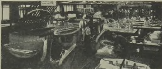
Forming of "Perspex" nose, canopies, etc., for the Halifax bomber at the Preston works
