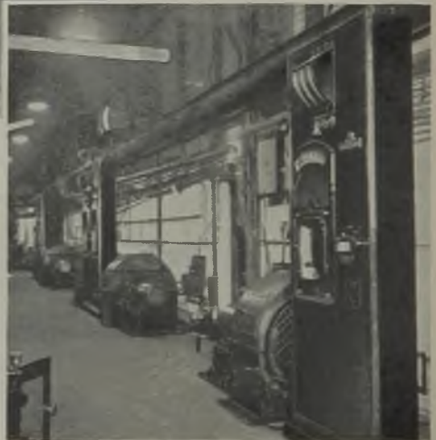
Above: The boiler houses are not merely parts of the power stations as is normally the case; five 16,000-lb. per hr. units
