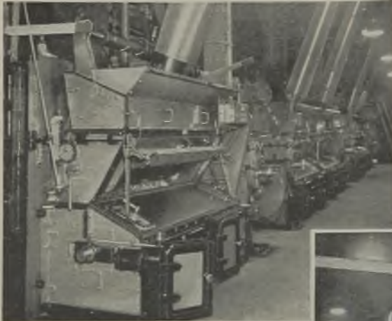
Above: The boiler houses are not merely parts of the power stations as is normally the case; five 16,000-lb. per hr. units
