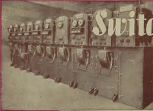
A ring main circuit breaker unit.
