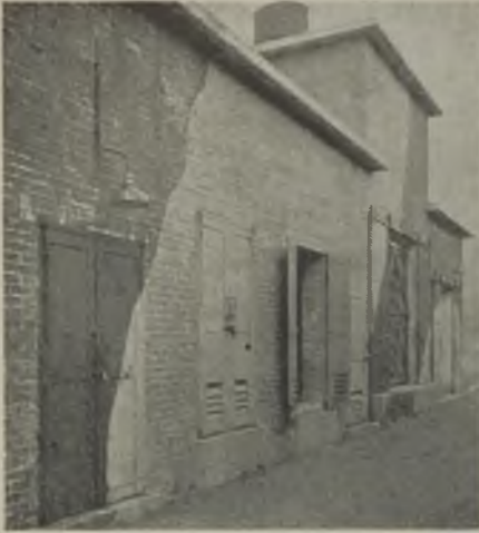
Each bulk-supply substation has separate compartments for, inter alia , the 33-kV switch (right) and the 6.6-kV switchgear (below); metering is effected at 6.6 kV
