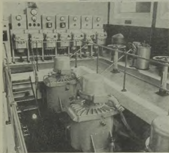
The water supply is of special significance; it is obtained from a pumping station about four miles from the factory
