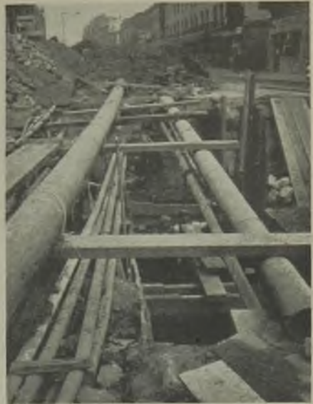
Repair work in progress near Cadby Hall, Hammersmith
