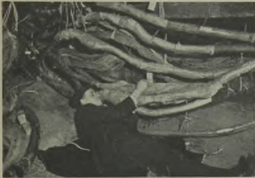
Repairing damaged cables at the Bishopsgate exchange, London
