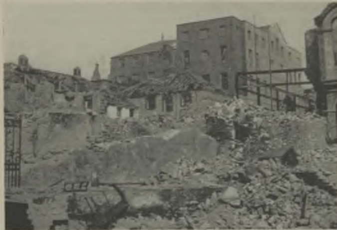
Plymouth telephone exchange
