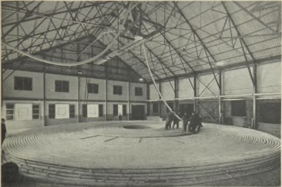
Special building erected by Siemens for coiling long lengths of the cable and special coiling gear
