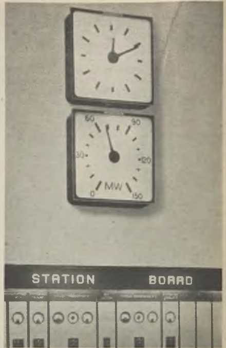
Fig. 3.—Megawattmeter (4 ft.) at Llynfi surmounted by station clock
