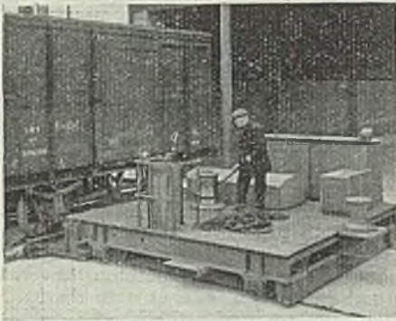
An electrically-driven wagon traverser in operation
