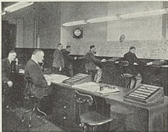
General view of the Stoke-on-Trent control room
