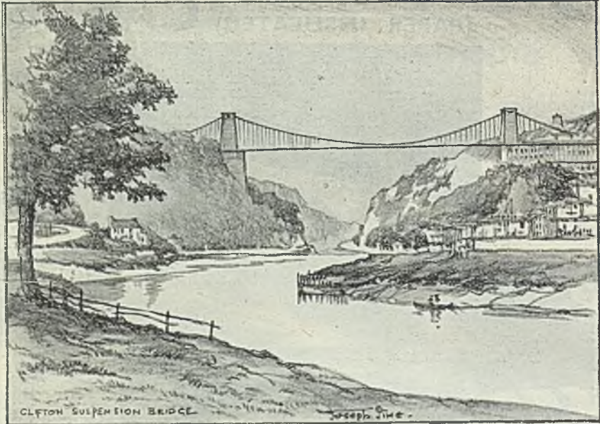
Bristol CLIFTON SUSPENSION BRIDGE Bridge 702 feet long from pier to pier. Spans the river Avon at a height of 245 feet. Completed 1864
