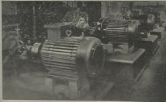
L.D.C. Flameproof Motors (Buxton Certified) Driving Benzol Pumps
