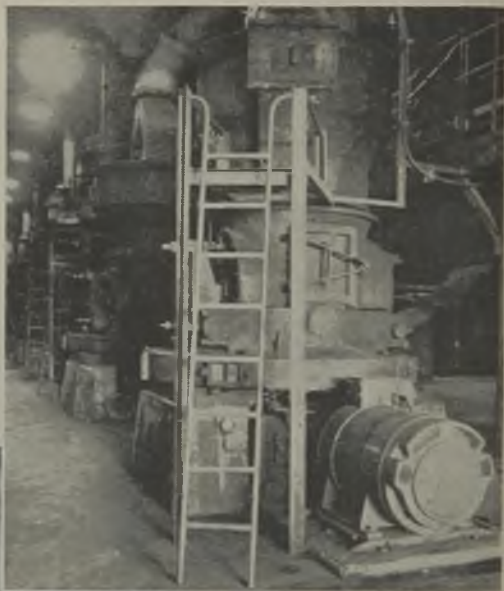
Above : The boilers are served by roller-type p.f. mills on the direct principle; two mills per boiler
