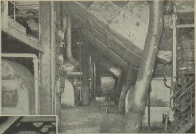
The rotary air preheaters (right) are located at the firing-floor level and face the feeder ends of the boilers
