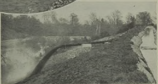
An extremely interesting point about the ash-disposal scheme is its possible influence, in relation to other factors, on the adoption of p.f. firing; ashes and water being pumped into the impound area
