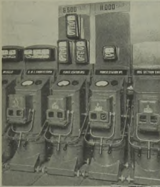
Above: Some of the 6.6-kV switch-gear at Harrowden has been "upgraded" to 11 kV
