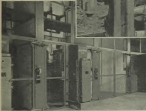
Burnt-out rotary converters and transformers at the Streatham substation and (left) the new 33-kV switchgear at the Purley substation
