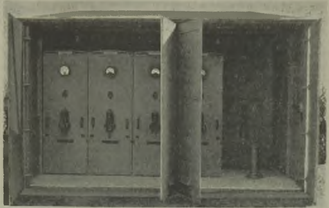
B.T.H. cubicle gear installed at Deadman's Cross to replace pole-mounted air-break gear
