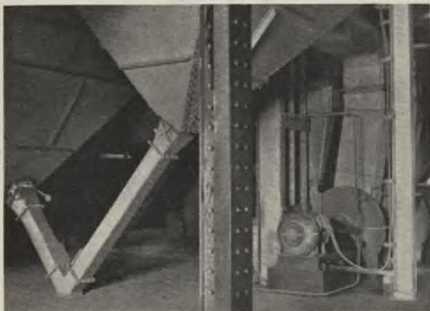
Secondary air fans are housed at basement level; ash and riddlings from the grates are fed into troughs under the basement floor
