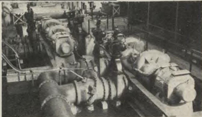
Circulating-water pumps each with a capacity of 924,000 g.p.h.
