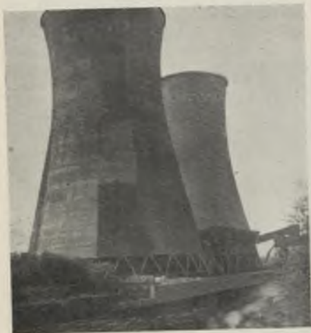
Two natural-draught hyperbolic cooling towers each deal with 1,850,000 gal. per hour
