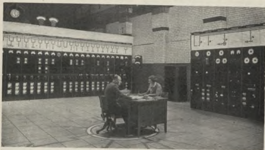
Switchgear is remotely solenoid operated from a spacious new control room
