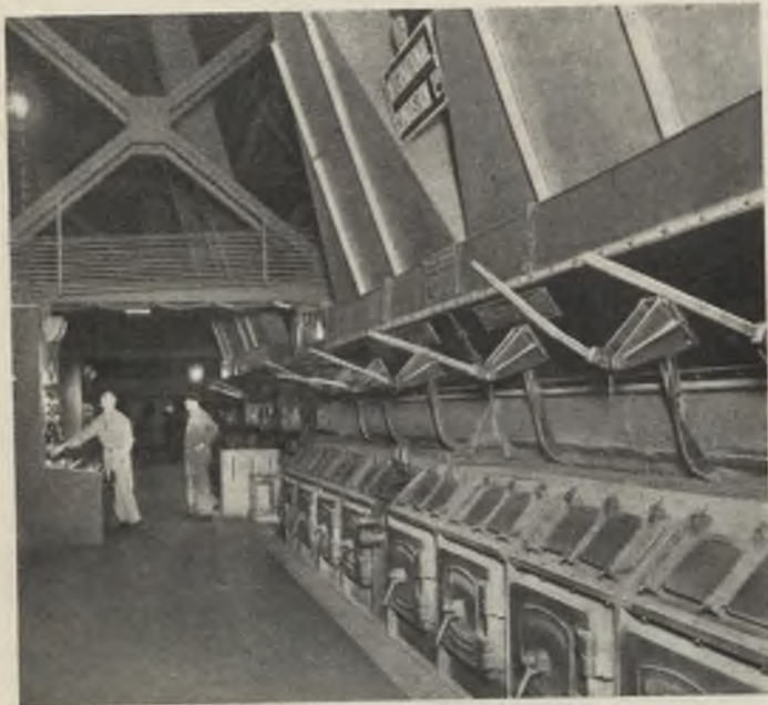
The five new boilers are now in a new building in two facing rows, with an unusually wide firing aisle
