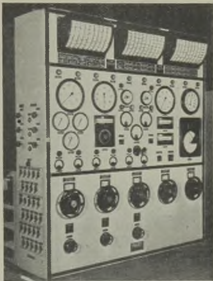
Control board for a large boiler operated with unified control
