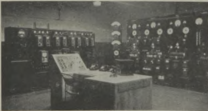
The main switchgear is remotely controlled from a central control room in which there are a separate four-panel board for each set and a grid metering board
