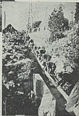
Underground Cable link to Overhead Line
