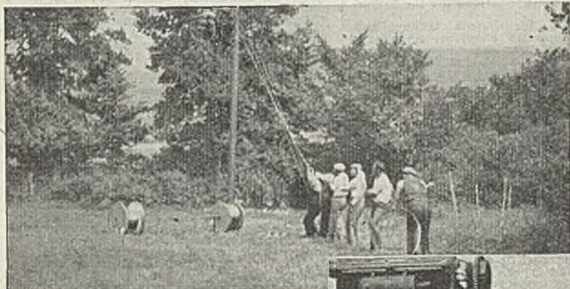
Overhead line in course of erection
