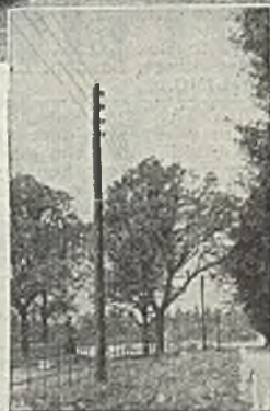
Completed overhead line
