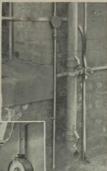
Earthing tails are brought out to the external base conductor; risers from earthing point
