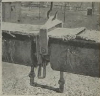
Coupling of flanges of T.N.T. overhead duct
