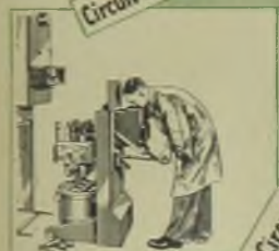
Circuit Breaker Truck withdrawn from cubicle
