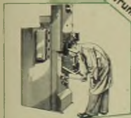
Circuit Breaker being racked down for isolation
