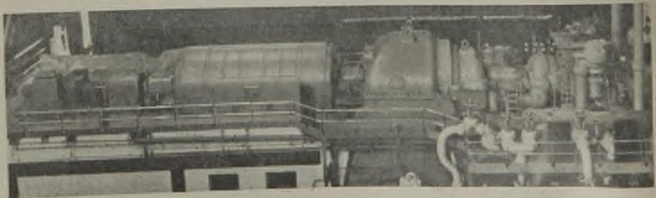
The 50,000-kW set has h.p. and l.p. cylinders and main and auxiliary alternators in tandem
