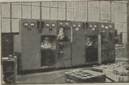
Typical large Hewittic Rectifier for mass charging of batteries
