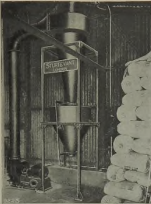
Sturtevant T.L. Cyclone on a rotary dryer
