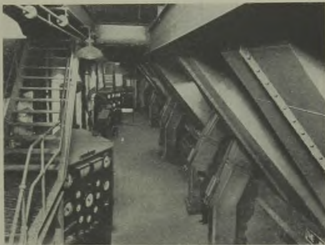
Four new 120,000-lb. per hour boilers have replaced six 40,000-lb. per hour units
