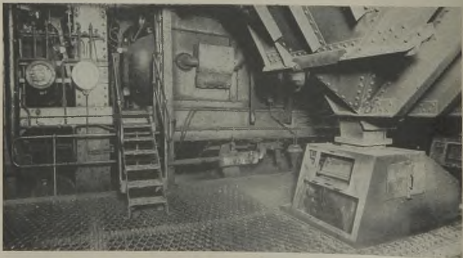
Each boiler has one forged steam and water drum, with riveted ends (left); automatic coal weigher (right)
