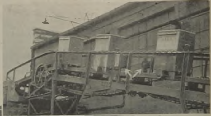
Above: On the first conveyor section the bins pass photo-electric cell equipment (indicated by arrows); guard removed for photograph Left: From the bins the non-ferrous metals are bagged and put on to a slat conveyor
