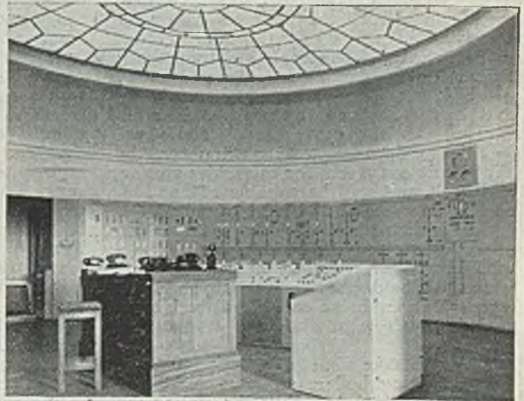
The control room
