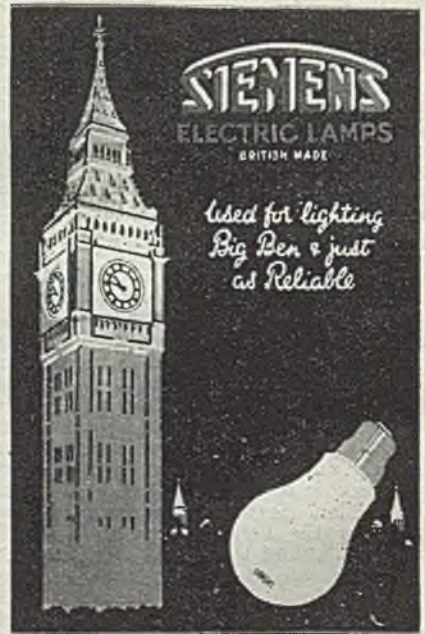
A striking Siemens' hanging display
