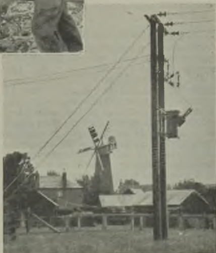
To reduce initial cost single-phase supplies are given to a number of hamlets, with provision for conversion to 3-phase later on. Above is a pole-mounted transformer stepping down the 11-kV, 3-phase supply to 230 V, single-phase, to serve Gedney Dyke
