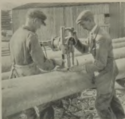
An electric groover in use on a pole for the G.P.O. at Calders Timber Works
