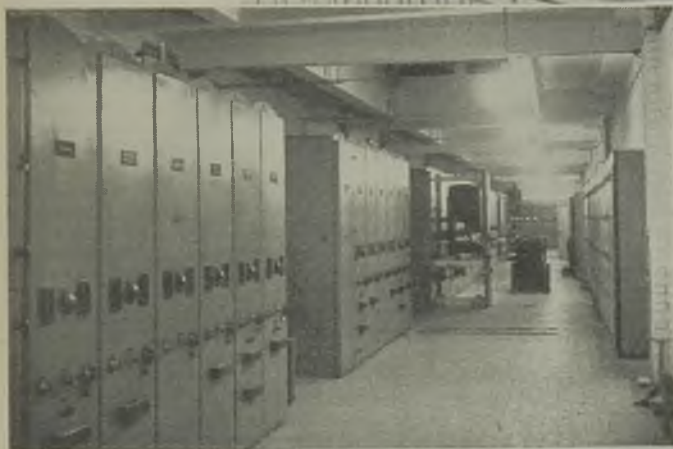
Only two sections of the whole station are separately housed — the auxiliaries switchgear (shown) and the p.f. mills
