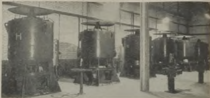
The centrifugal vertical circulating pumps are driven by 265-HP direct-starting motors
