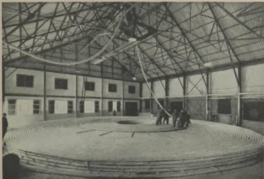
Coiling 40 miles of "Hais" Cable
