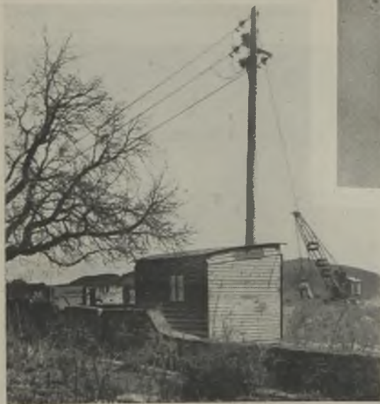
The 3-kV transmission is extended southwards from the cables by means of an overhead line
