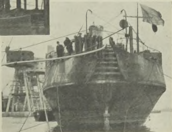
Above: Overhead catenary carrying the cable direct from the factory to the laying vessel.
