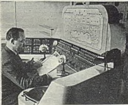
Control console of the public address system at Butlin's holiday camp at Filey
