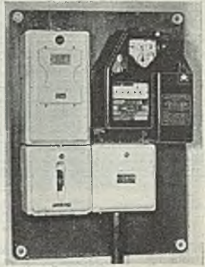
The unit in a similar recess, with sunk wiring and back-connection box
