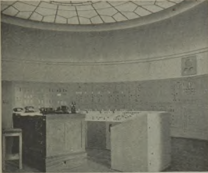
Main control room
