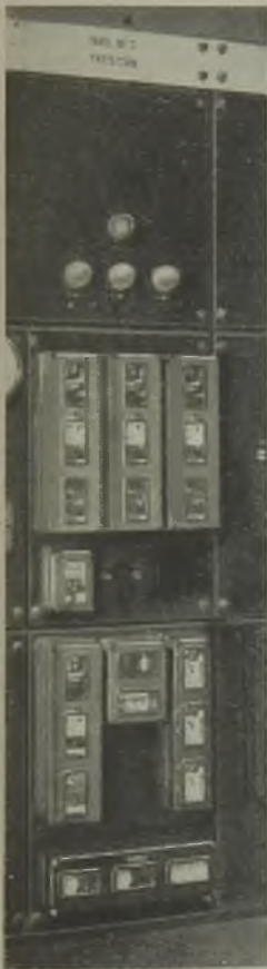
Fig. 5. — Typical assembly of relays on self-contained cubicle
