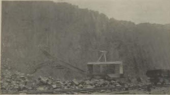
All-electric excavator at rock face of Hillhouse Quarries, the first industrial consumer of the Board
