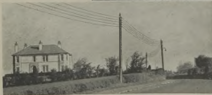
A good example of five-wire vertical-formation low-voltage distribution is that at Fenwick
