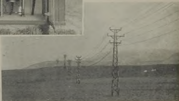
An exception to the general 11-kV line construction scheme is the double-circuit line from West Kilbride to Largs which has steel lattice masts
