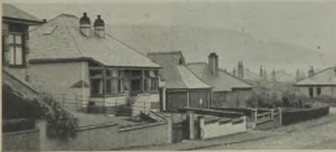
Residential area substation at Largs designed to preserve the amenities of the district
