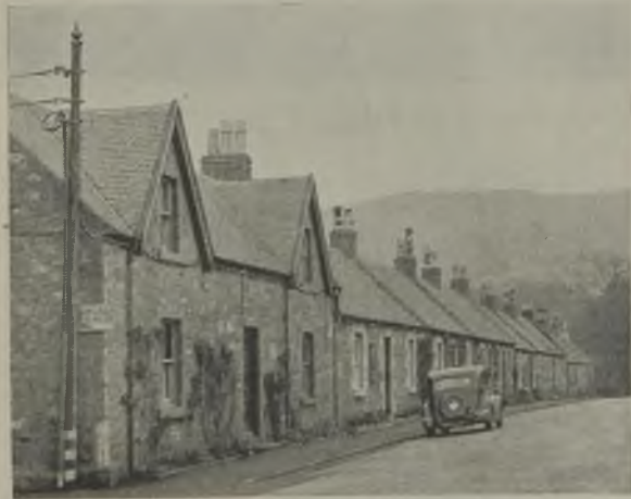
An excellent scheme to preserve local amenities is the low-voltage distribution at Straiton; special cable under the eaves of the buildings
