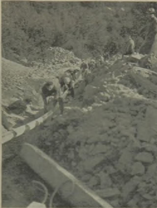
(3-core 66 kV cable being laid in difficult country).
