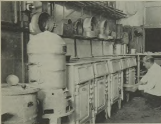
Domestic type cookers are used to good effect in the all-electric canteen of the North Western Engineering Co.
