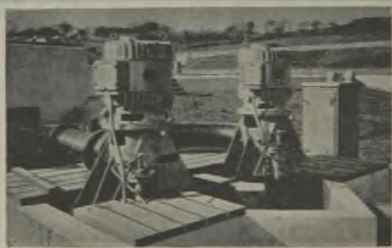
L.D.C. Weather-proof Motors, operating in the open, driving Sludge Pumps.
