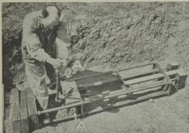
Thrust borer in entry pit beside 25-ft. concrete roadway
