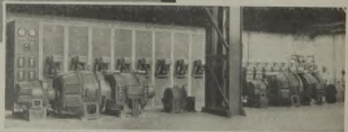
The boilers are stoker fired, each unit being equipped with twin travelling chain-grate stokers. Combustion is controlled by the unified system of control; two m.g. sets and switchboards (right)
