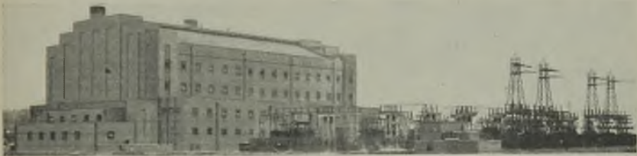
Mexborough is a riverside-operated station and it is being completed in its initial stage with its full plant capacity of 60,000 kW
