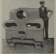
Illustration shows— "COG WHEEL" BRAND Phosphor Bronze Pump Body Casting for Sagar MIL. Weight - 3619 lbs.
