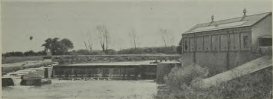
The small hydro-electric station at Linton-on-Ouse makes a useful contribution towards meeting the fuel shortage
