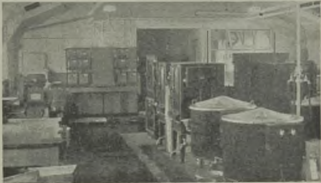
Some of the electrical equipment at the Harwich central kitchen for school meals
