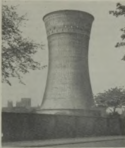
Though criticised the Electricity Department's new cooling tower is a graceful structure
