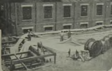
Cabling at Southwick Generating Station.
