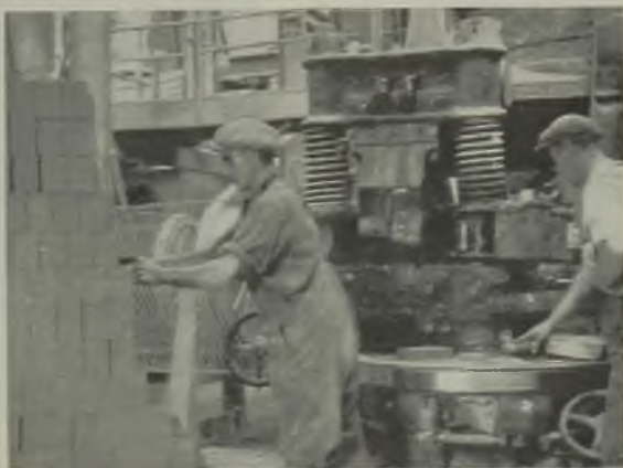
Making sand and lime bricks at John Laing's Calsil Brickworks
