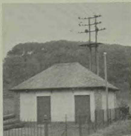
Typical brick-built substation at Bampton, with one of the few sections of overhead lines
