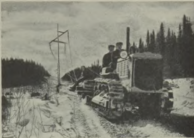
The stringing of power conductors in the rough northern districts of Ontario is facilitated by caterpillar tractors
