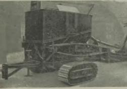
by the well-known "Colcrete" process. It is pumped from the mixer direct into the grout car (fig. 7) which is then hauled by a tractor and coupled to the plough by a simple tow bar. Inside the grout car tank a catherine wheel rotates in bearings, one of which can be seen about half way up the tank.
