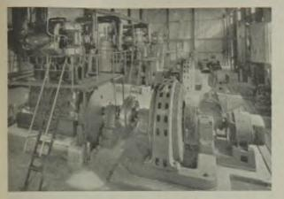
General view from air-intake side showing compressors, autosynchronous motors and starting gear
