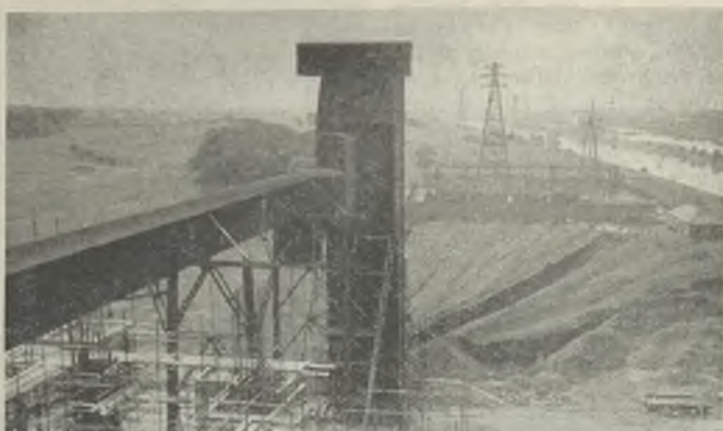
On the west side of the station a conveyor links with a tower at the edge of the storage ground
