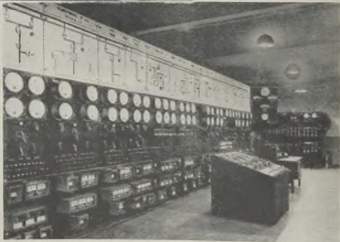
Switchgear "A" is remotely operated from the control room in the old generating station
