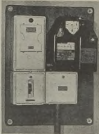
The standard unit with sunk wiring and back connection box.
