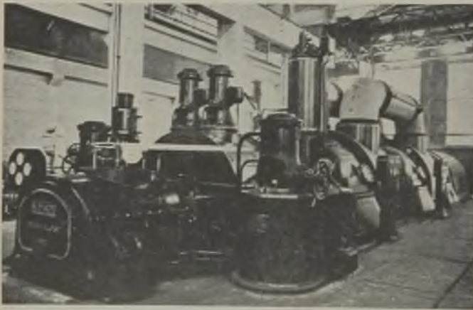
Generating plant at St. Denis
