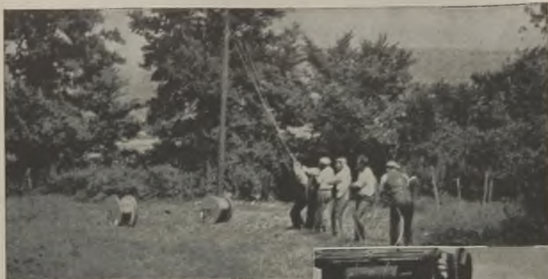
Overhead line in course of erection
