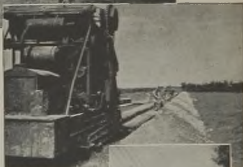
Mechanical excavation of cable trench
