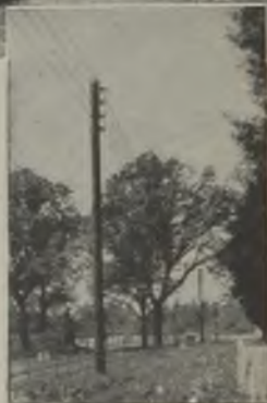
Completed overhead line
