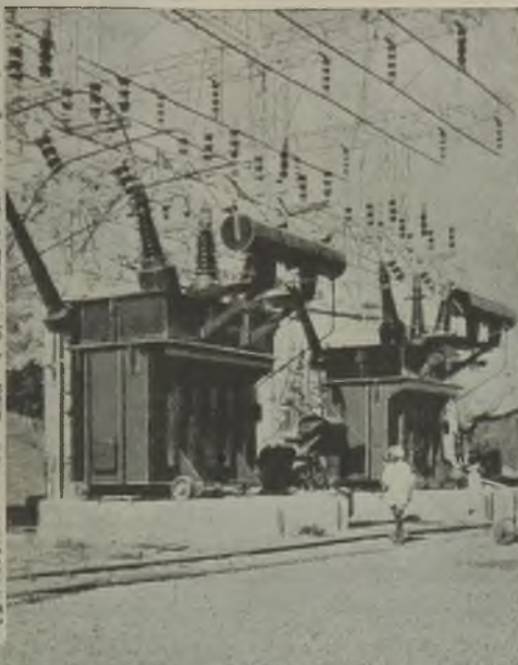
Left: A "Metrovick" 110 kV 3-phase outdoor transformer at a power station in Madras,
