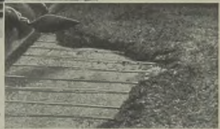
The 12,000-egg incubator with transformer and control gear on the left, and (right) a 2 in. layer of cement and sand being placed over the iron wires
