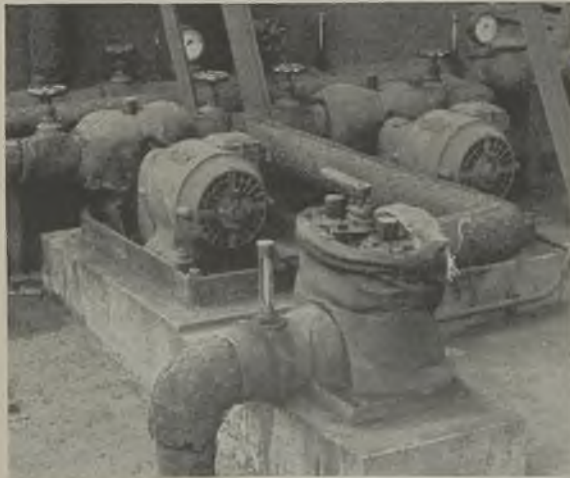
The hot fuel is pumped from the storage tanks by motor-driven units integral with the system
