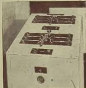
A typical multi-facility panel
