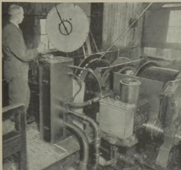
Above: The double-drum winder is driven by a 120-HP motor with double spur gear transmission
