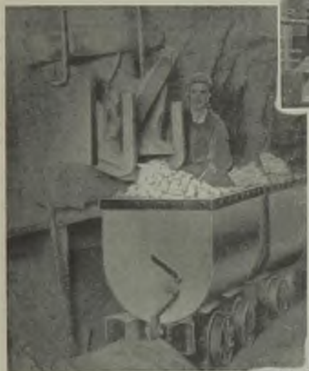
Limestone mined from the Halkyn mountain is fed from the stope down the vertical chutes at the bottom of which it is collected in the cars (centre). Trains of cars are hauled to the shaft bottom by electric locomotives (right)
