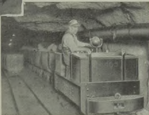
Limestone mined from the Halkyn mountain is fed from the stope down the vertical chutes at the bottom of which it is collected in the cars (centre). Trains of cars are hauled to the shaft bottom by electric locomotives (right)
