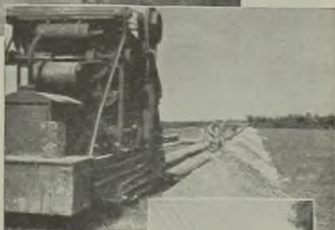
Mechanical excavation of cable trench
