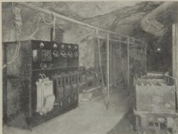
Adequate arrangements are provided for charging the locomotive batteries underground
