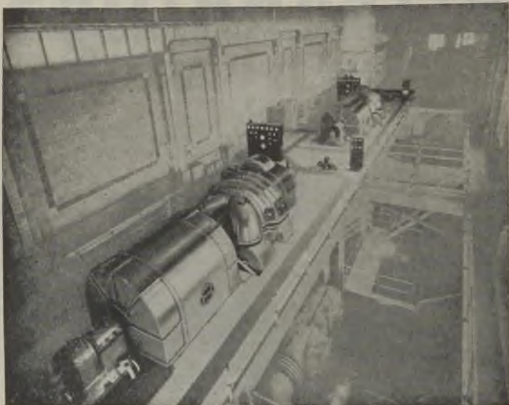
Two 15,000 kW. Parsons Turbo-Alternators supplied to the Corporation of the City of Edmonton, Alberta, Canada.
