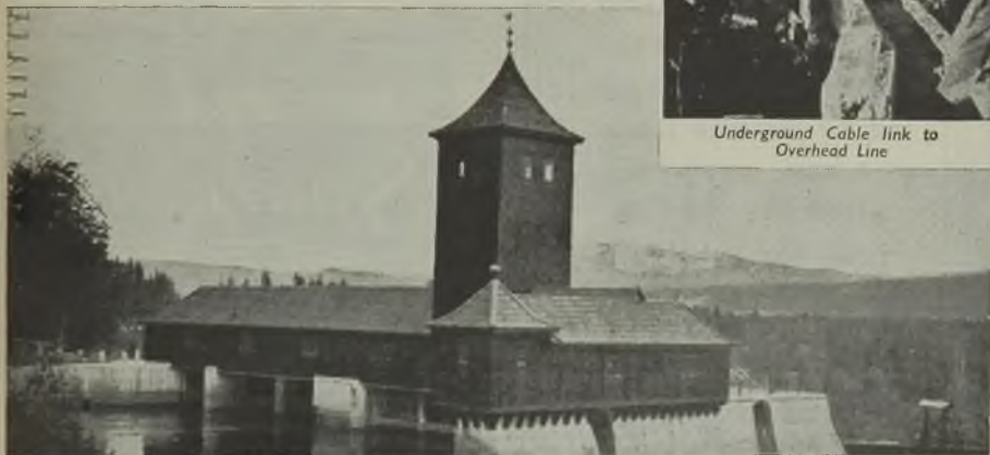
Hydro-electric Generating Station
