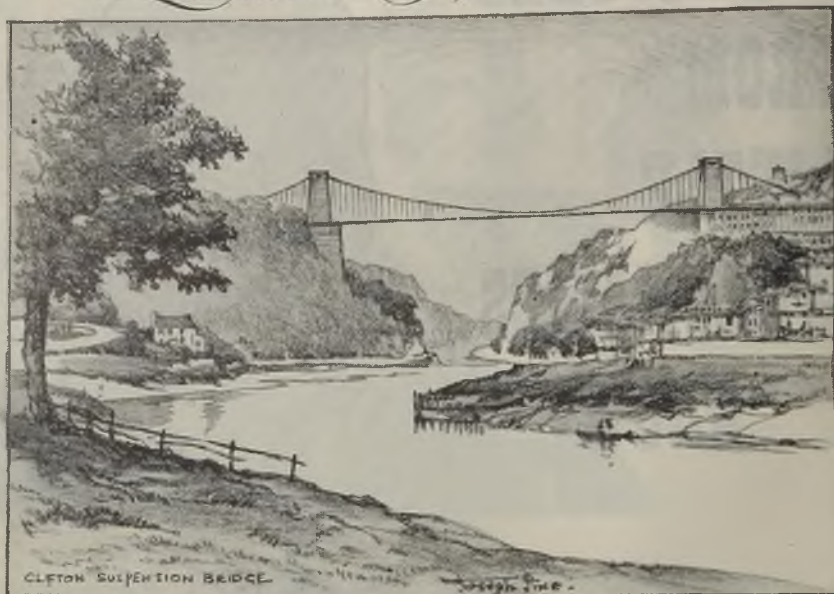
CLIFTON SUSPENSION BRIDGE
