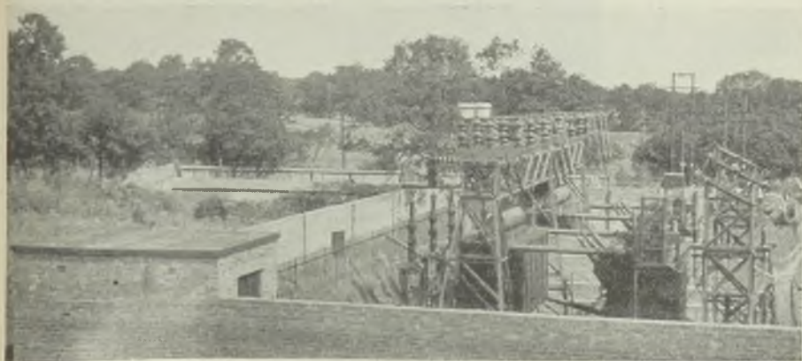
The 66/33-kV transformers at Legacy receive from Maentwrog via the main system 66-kV interconnector
