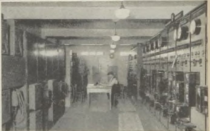
The Hawarden substation can be brought completely under the supervision and control of the Legacy control room. The Hawarden control room (right) houses vertical remote control panels in addition to supervisory equipment
