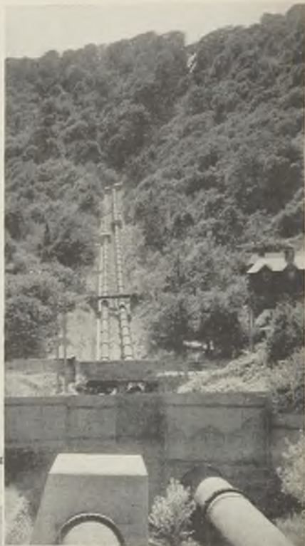
The Dolgarrog power station operates with an effective full head of 1,150 ft.; lower pipe-lines on 500 lb. per sq. in. pressure
