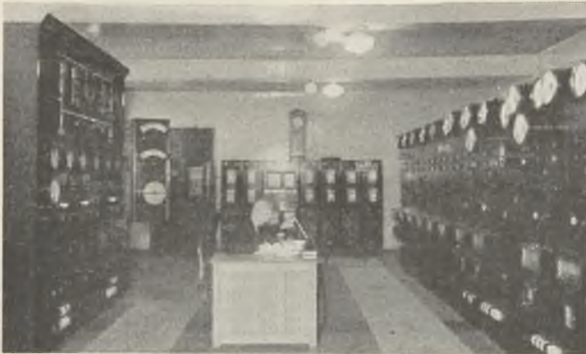
Remote switching of the 132-kV equipment in the C.E.B. substation and the power company's 33-kV switches is effected at the Crewe control room
