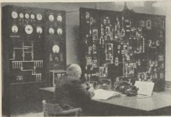
The Hawarden substation can be brought completely under the supervision and control of the Legacy control room. The Hawarden control room (right) houses vertical remote control panels in addition to supervisory equipment
