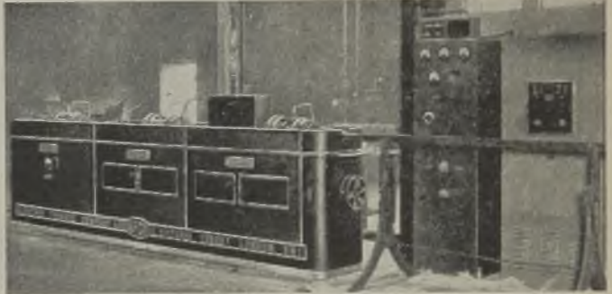
At No. 3 station (induction heating) the bar passes slowly through a multi-turn coil
